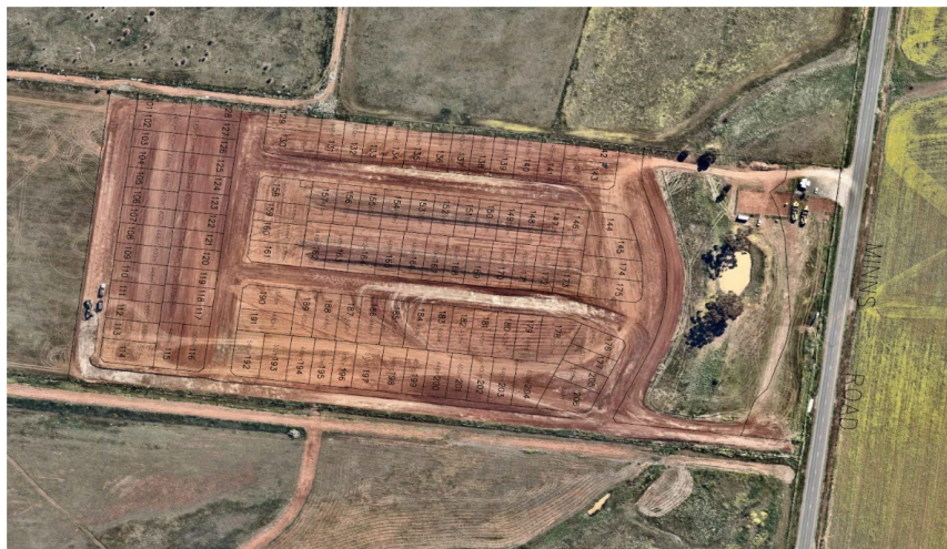
Image: 413-439 Minns Road – Project view during construction.
