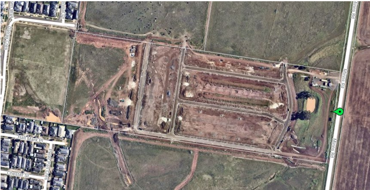
Image:413 Minns Road, Kurunjang – Project view toward completion.
